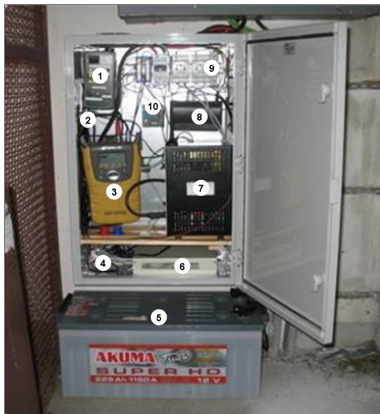
Fig. 3 Configuration and equipment of the GEONAS stations. 1 - main power supply, 2 - GPRS modem, 3 - GNSS receiver Topcon GB-1000, 4 - ethernet switch, 5 - battery 225 Ah, 6 - minicomputer for data pre-processing (processor VORTEX86/166 MHz, 40GB HDD or CF 32GB, Debian GNU/Linux), 7 - battery charger, 8 - ethernet switch 100 Mbit/s, 9 - undervoltage protection, 10 - cooling system
